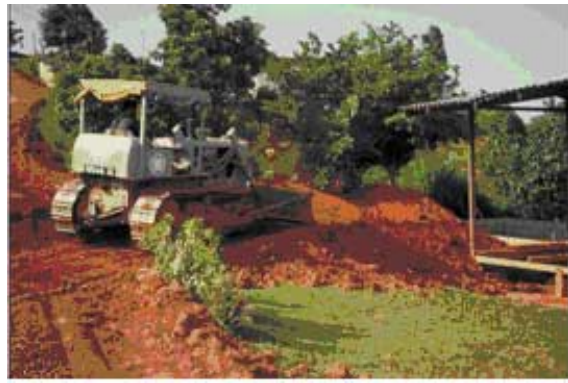
Figure 8: Cutting a New Road
