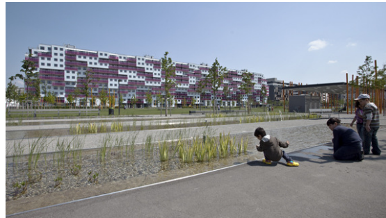
Figure 8: Bednar-Park and Housing complex
