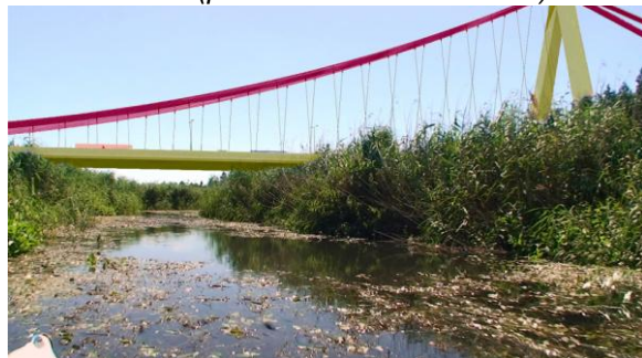
Fig. 11. The approximate view of assumed suspension bridge II (80 m height) from about 200 m (photo Zb. M. Michniowski)
