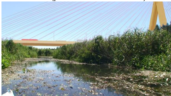
Fig. 8. The approximate view of assumed suspension bridge I (120 m height) from about 200 m (photo Zb. M. Michniowski)
