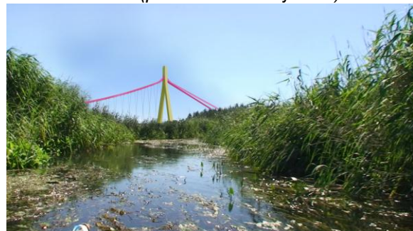
Fig. 10. The approximate view of assumed suspension bridge II (80 m height) from about 400 m (photo Zb. M. Michniowski)
