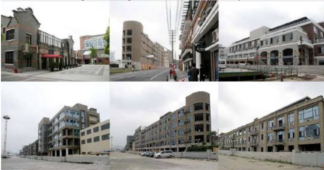
Figure 15: Photos of present reconstruction (May 2010)
