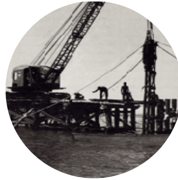
Figure 2. Workers on a dock
