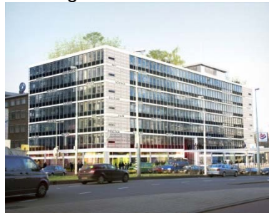
Figure: Schieblock Rotterdam NL
