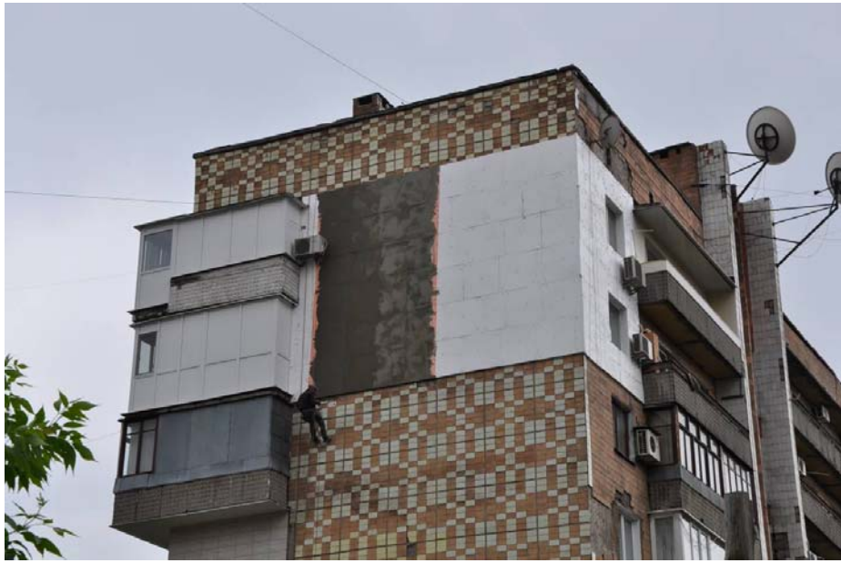
Figure 3: Single insulation activity for two apartments
