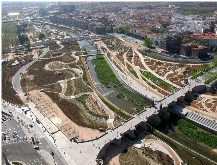
Figure 2: Surface space freed up by placing the M30 motorway underground in Madrid ©Municipality of Madrid
