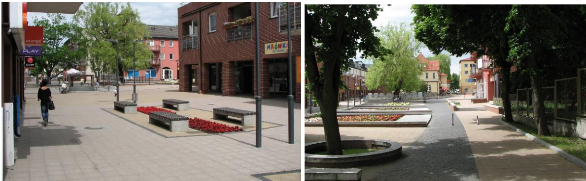
Fig. 4-5. New town center in Pruszcz Gdański.
