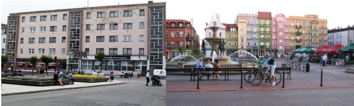
Fig. 8. The Old Market Square before renewal (source: Municipality of Chojnice).
