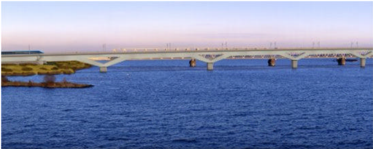
Figure 2 the Hollandsch Diep Bridge. Source: www.hslzuid.com
