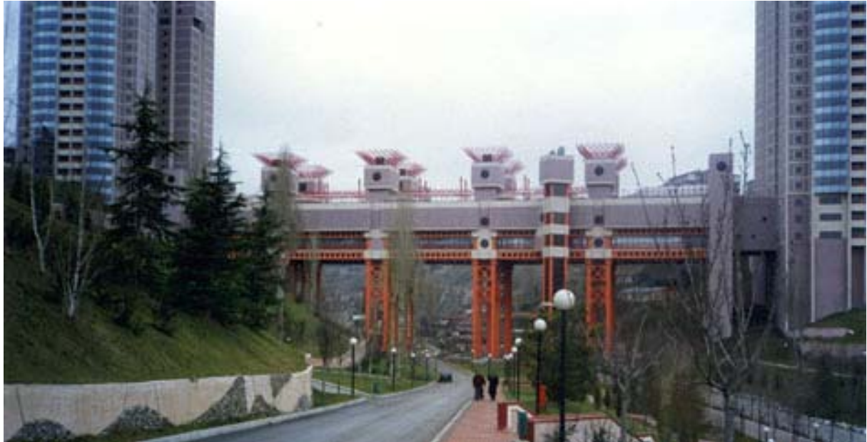
Dikmen Valley, 1998: the two 30 floors 'twin towers' and the connecting bridge built across the valley are being accomplished.
