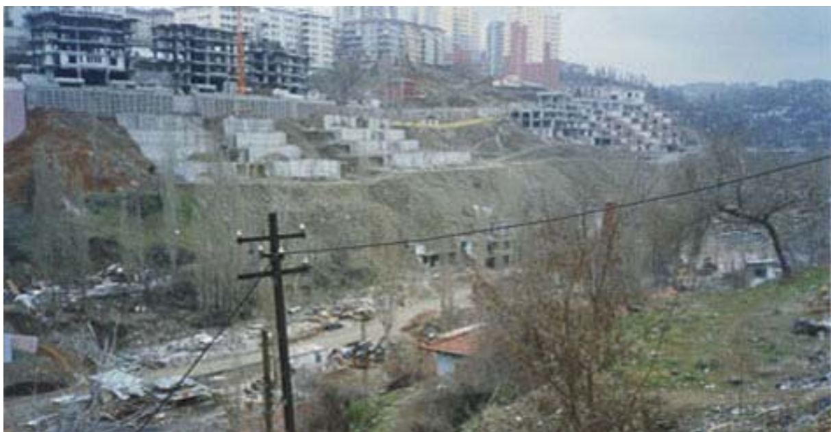
Dikmen Valley, 1998: Dikmen Park works starting and new houses under construction on the hill.
