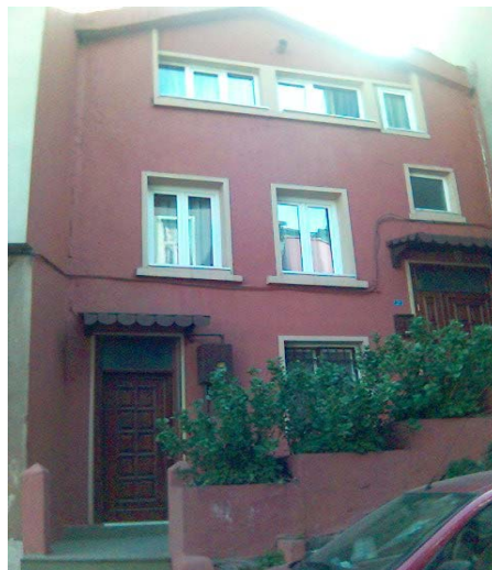
Photograph 8; A Rehabilitated building from Visnezade Neighbourhood Source: Photographs taken by one of the authors Hurrem Betul Levent
