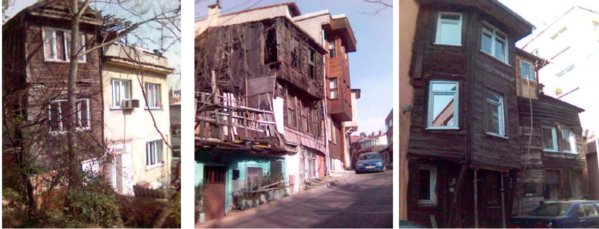
Photograph 1,2,3; Historical Demolished Wooden Houses of Visnezade Neighbourhood
