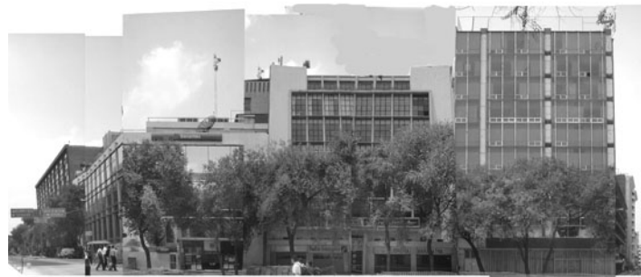
8. Citibank-Banamex – Private building – Light Co. building
