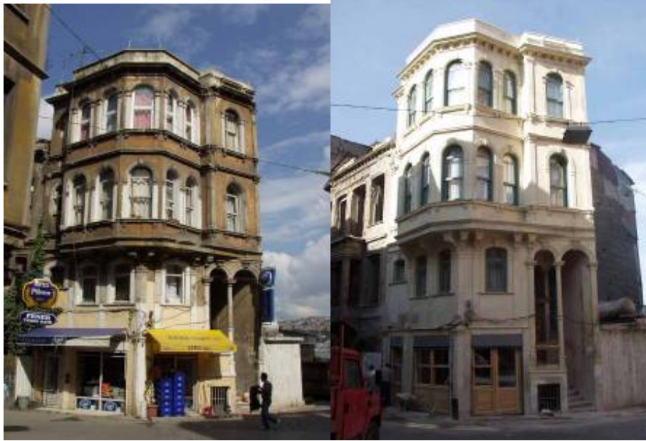
PHOTO 4-5. TEVKII CAFER QUARTER, VODINA STREET, NO: 2 (BEFORE AND AFTER RESTORATION)
