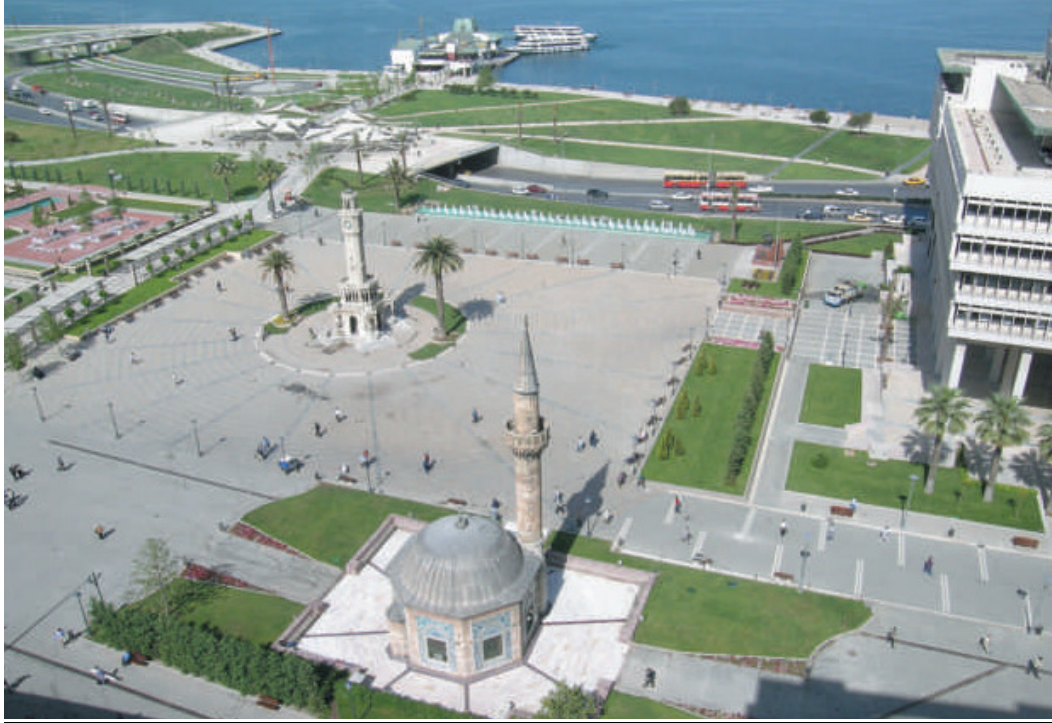
Figure 1 View of Konak Square, Source: Ege Mimarlik 2004/2-50 p.52
