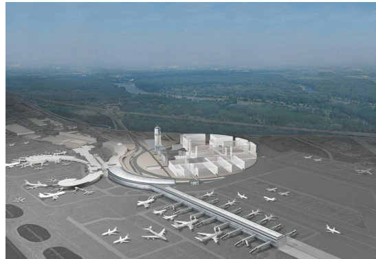
"Sky-Link" and Officepark at Vienna International Airport (currently under construction)
