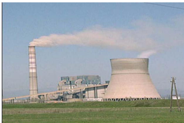
Figure. 8. Thermo Power Plant,- Kosova B.
