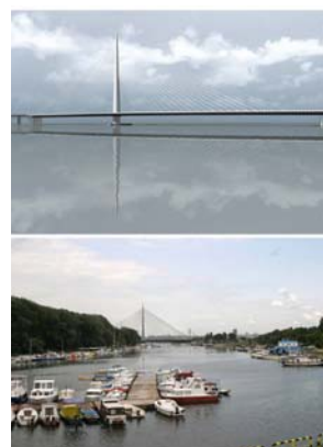
figure 3. New bridge on Sava River, NBG
