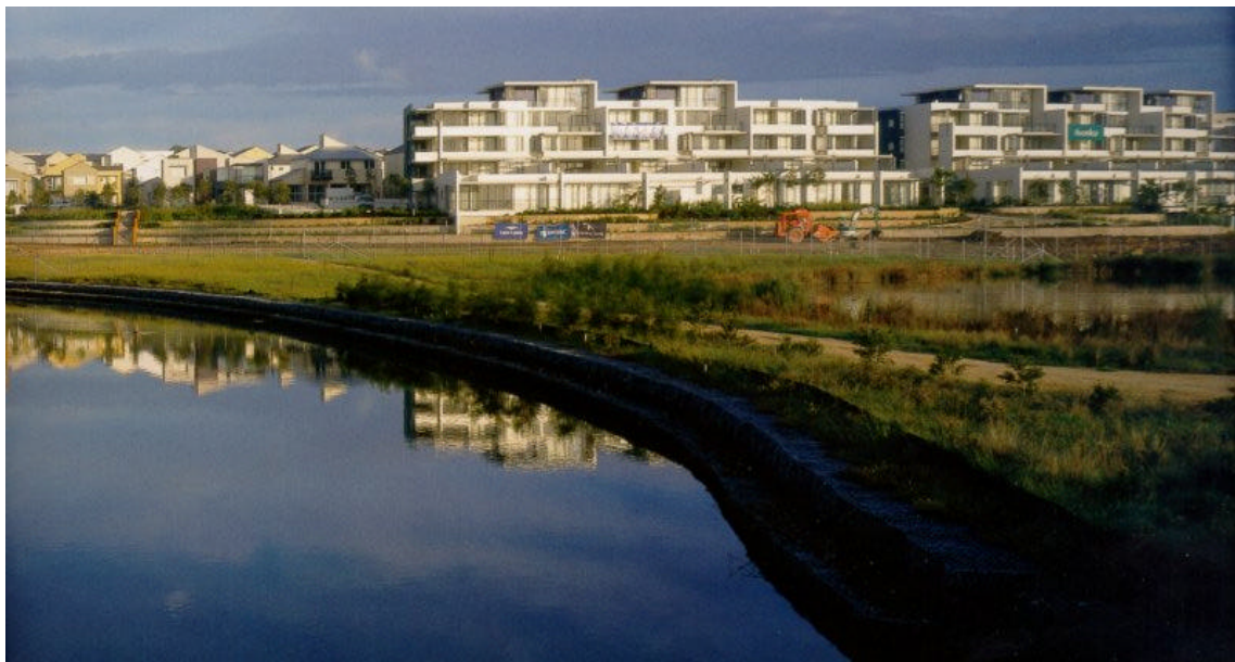
FIGURE 4 RESIDENCES CONSTRUCTED POST REMEDIATION
