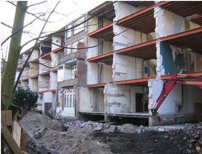
Construction; demolition of the back facades
