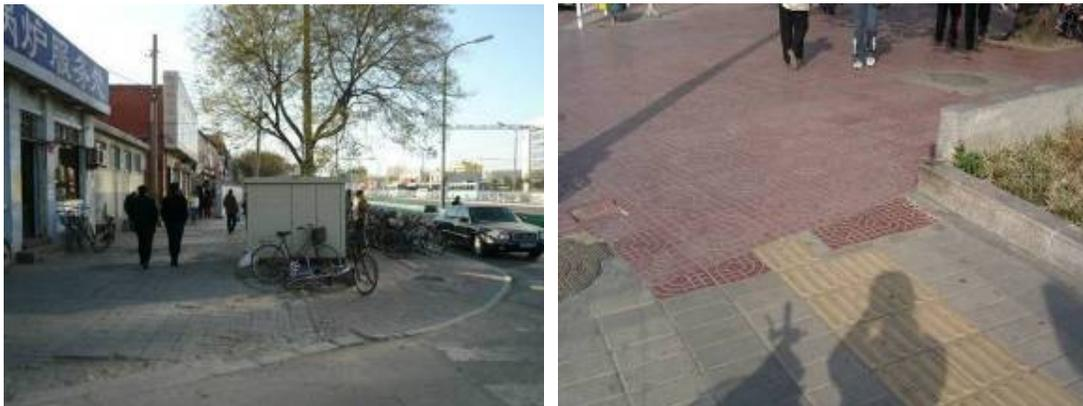
Figure 10~11. broken pavement and discontinuous blind lanes
