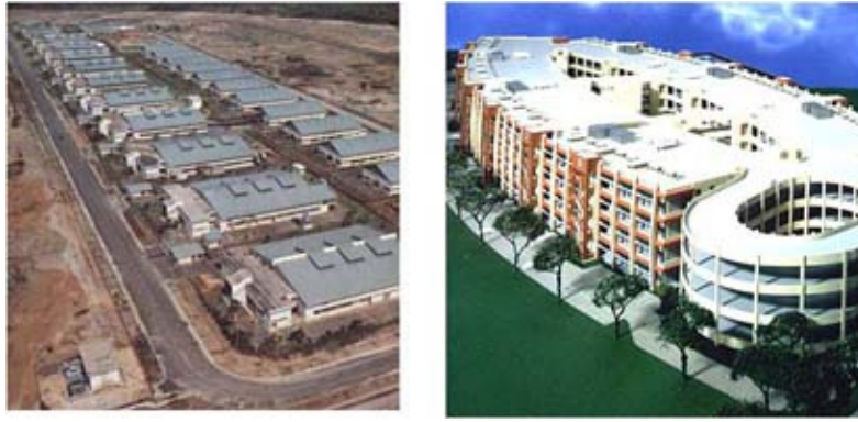
Figure 3: (left) Singapore's Jurong industrial area in the 1960s and 1970s was made up of large parcels of single-user, low intensity factories. (right) An example of Singapore's newer 7-storey ramp-up factories, with a ramp (right of picture) that allows container truck access and loading/unloading on every floor.
