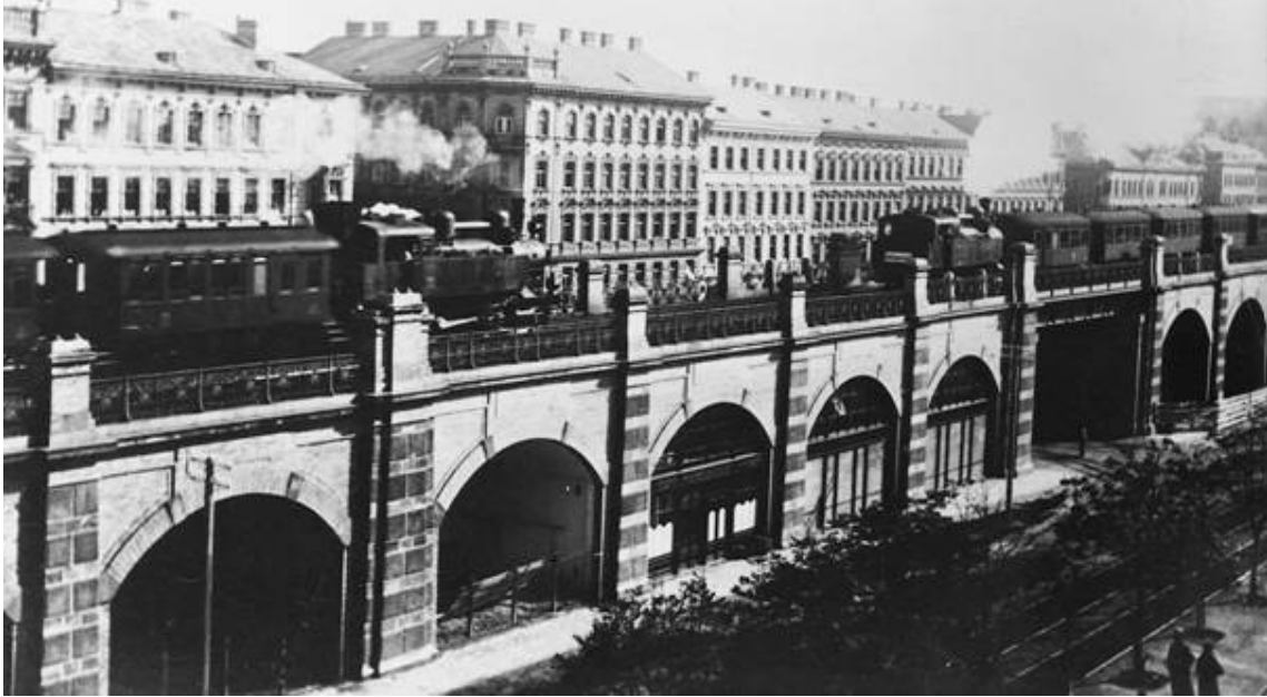
Fig. 3 The Stadtbahn viaduct was built in the center of the Gürtel Boulevard from 1893 -1898 and was constructed to support heavy loads, e.g. trains with steam powered locomotives.
