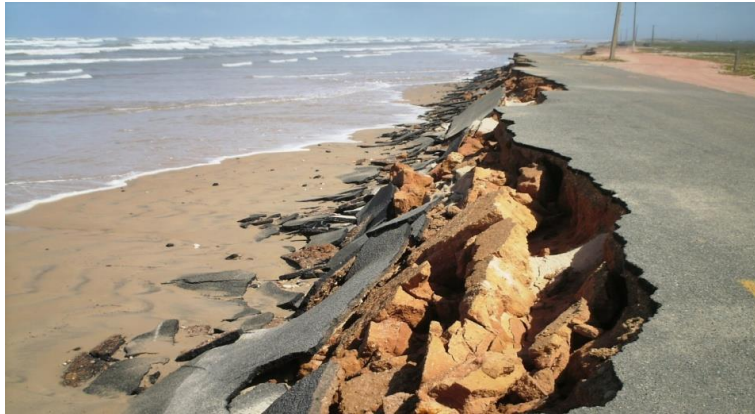
Figure 9: Destruction of the track that of the access to the lighthouse of the Mosqueiro. 2007/08/12.
