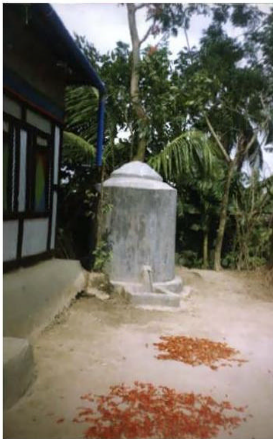
Photograph 02 (c): Rain Water Harvester.
