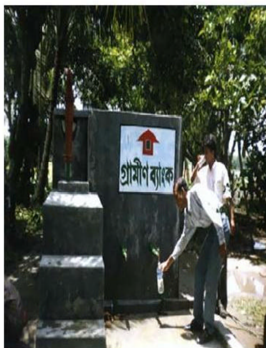
Photograph 08 (b): Pond Sand Filter.
