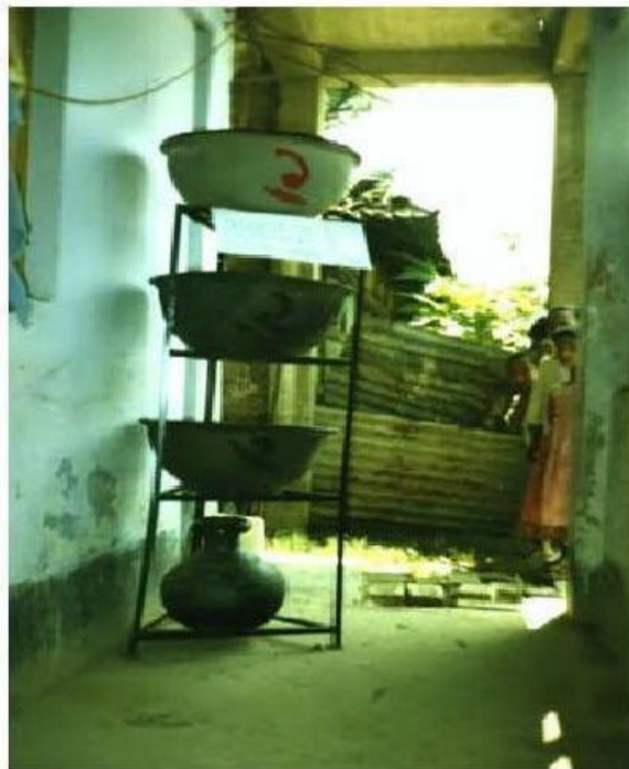
Photograph 07. (b): Bucket Filter.
