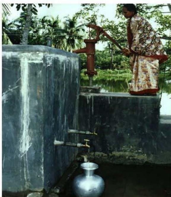
Photograph 08 (a): Pond Sand Filter.
