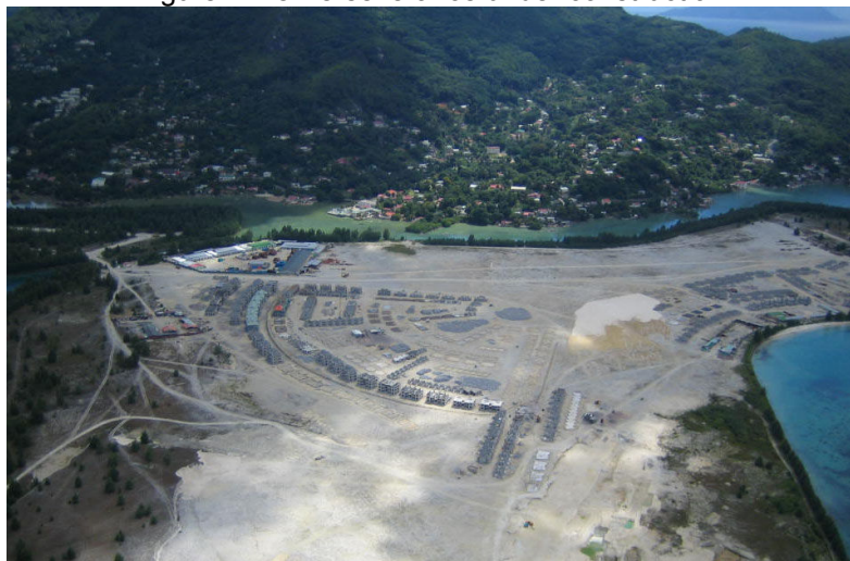
Figure 4- Ile Perseverance under construction
